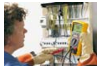
Insulation test at a distribution panel
