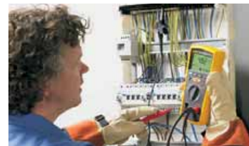
Insulation test at a distribution panel
